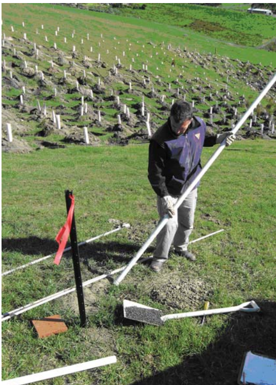
Figure 3. Dale Worledge installing a piezometer.
